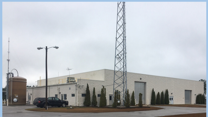
NC Dixon plant front
