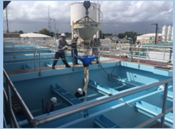
Figure 8: Rehabilitation of Media Filters
